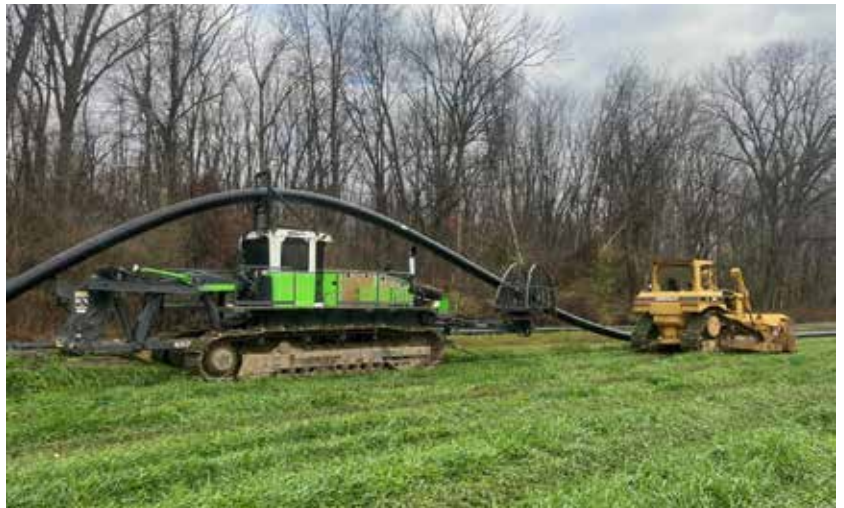
Photo: Manure transfer line being installed.
